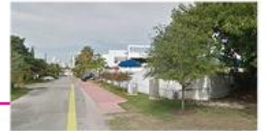
Lack of Sidewalks
