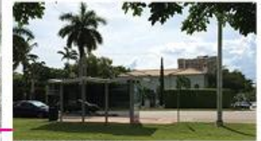
Existing Bus Stop
