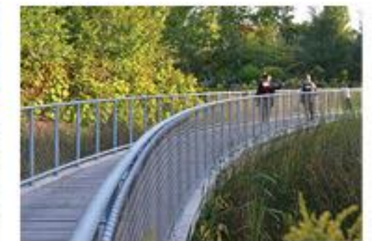
Recycled Plastic Planks & Metal Railing with Mesh
